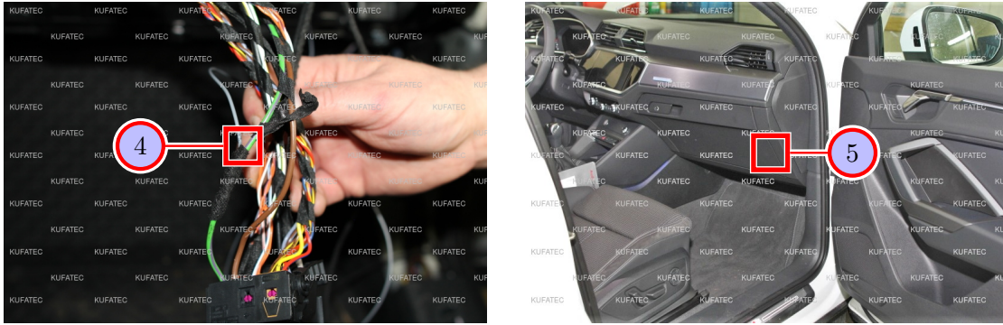
Figure 13: Connection cable set
